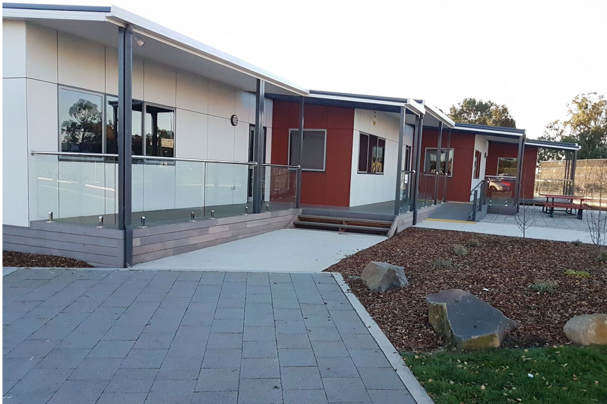
New Demountable Classrooms
